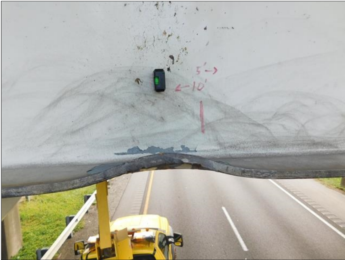
Span 2 Beam 1: Supplemental Inspection Impact Damage, Span 2 Beam 1 IS OUT OF PLUMB UP TO 5 Degrees EASTWARD AT Point of Impact WHICH IS 17 FOOT 2 INCH FROM Bent 2. IT IS OUT OF PLUMB FOR A TOTAL OF 15 FEET, 10 FOOT NORTH OF THE Point of Impact AND 5 FOOT TO THE SOUTH. (PAR)
