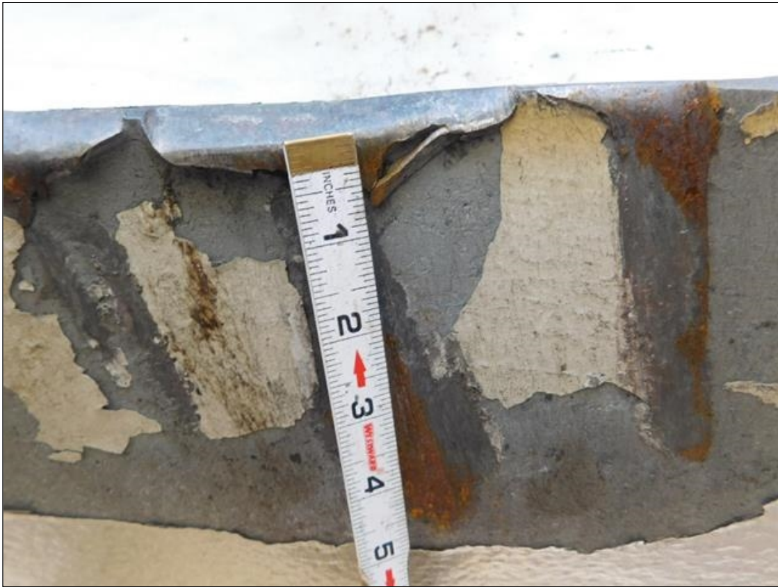
Span 2 Beam 1: SUPPLEMENTAL INSPECTION IMPACT DAMAGE, SPAN 2 BEAM 1 AT THE POINT OF IMPACT LOCATED 17 FOOT 2 INCH FROM BENT 2 THE BOTTOM FLANGE IS BENT UPWARD ON THE WEST SIDE. THIS IS 2 FOOT LONG X 2 INCH HIGH X 9 INCH ACROSS. THERE IS A 6.5 INCH LONG X UP TO 1/4 INCH DEEP X 5 INCH ACROSS GOUGE IN THE CENTER OF THE BENT BOTTOM FLANGE ON THE WEST SIDE. AT THE SAME LOCATION ON THE EAST SIDE THE BOTTOM FLANGE IS BENT DOWNWARD UP TO A 1/4 INCH OVER A 20 INCH LENGTH. (PAR)
